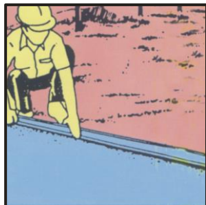
Evenly Spread the Layer of Sand over the Sub-base
