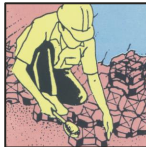
Lay and Interlock Paver Blocks
